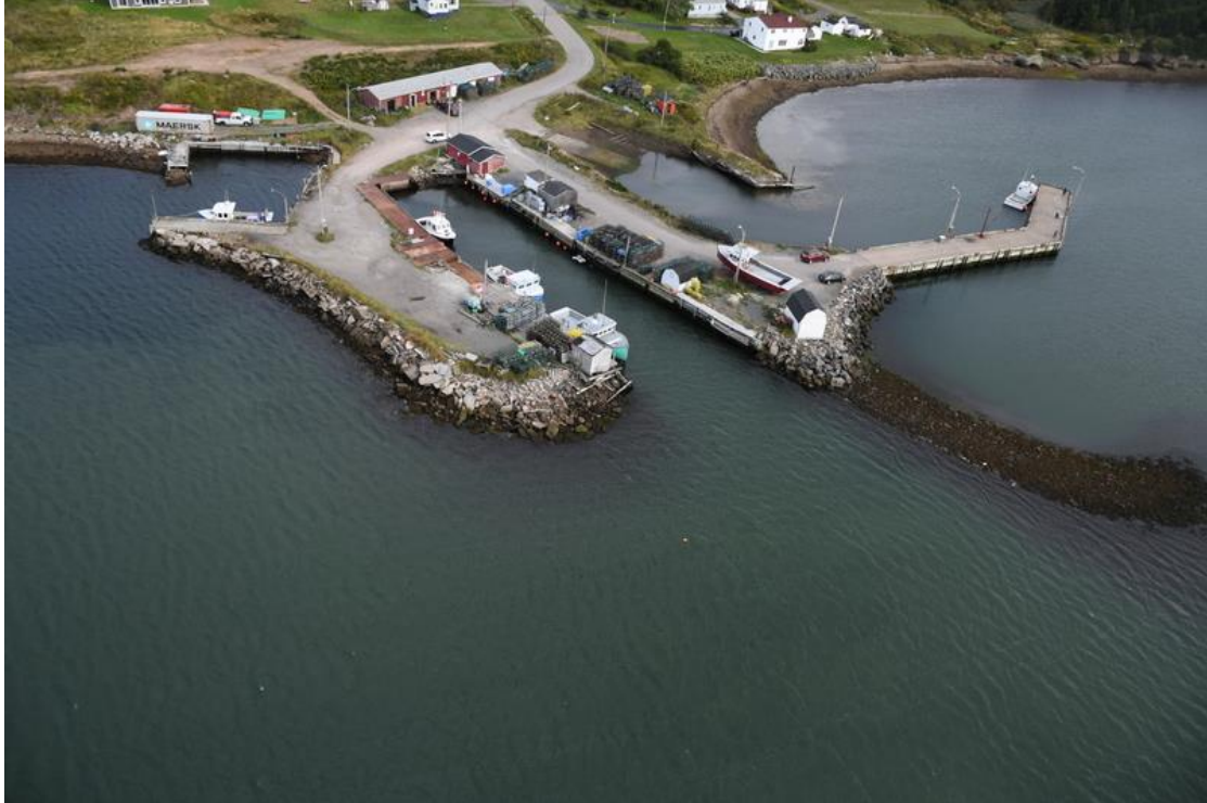
Photo ns22_sd_15726: Example of Coastal Class 32; Permeable man-made structures. South Bar.
