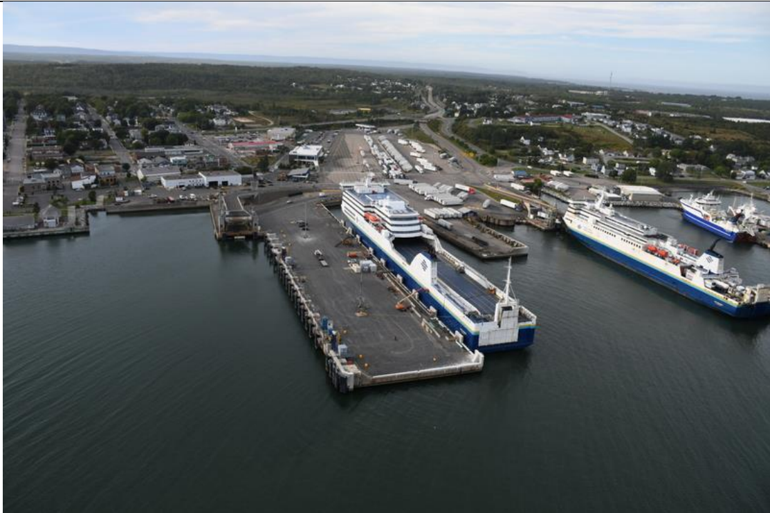
Photo ns22_sd_16668: Example of Coastal Class 33; Impermeable man-made structures. North Sydney.
