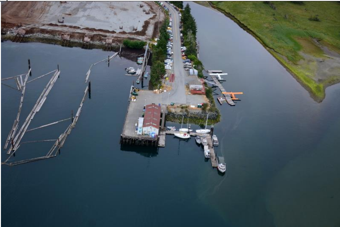
Photo bc21_nk_01772: Example of Coastal Class 32; Permeable man-made structures. Muchalet Inlet.
